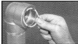
**2** Fitter seats ring into fitting. Spring tension holds ring tightly in place, assuring no rattling or vibration even under extreme pressure. Ring actually becomes a permanent part of the joint.
